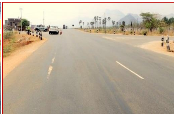
Typical intersection with no controls/signage (NH47 By-Pass, Vellalur junction)
