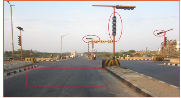
Non-functioning traffic signals in NH47-209 junction. Lack of lane markings and poor intersection alignment.
