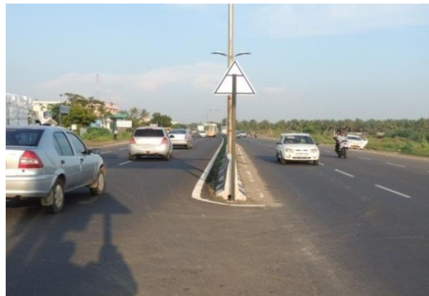
Vehicle movement on a median-separated road (NH47)
