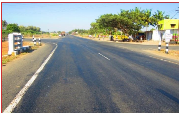
Typical intersection with no controls/signage (NH47 By-Pass, Pattanam Pudur junction)
