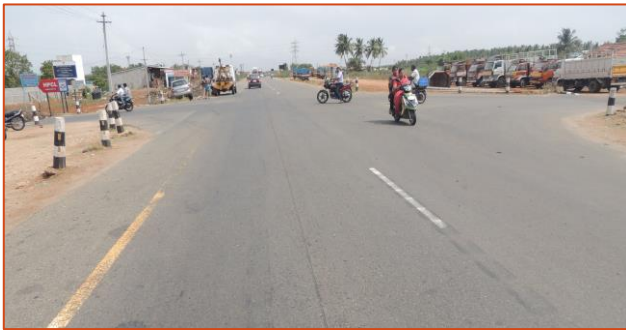
NH47 By-Pass, Irugur junction – no warning signs.
