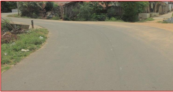
District road, Selvapuram
