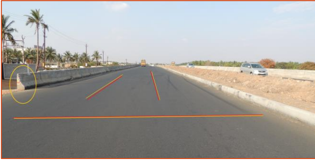
NH47 no lane markings - no warning signs of bridge wall.
