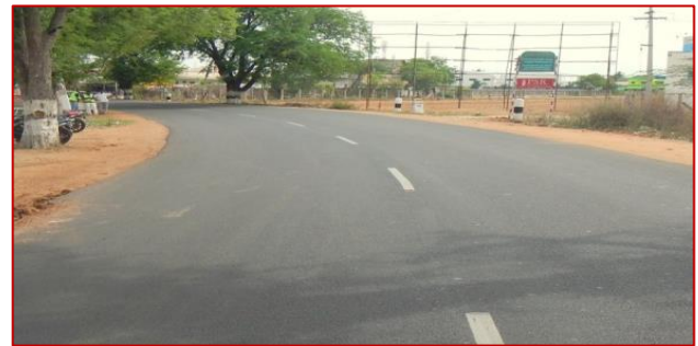
Undivided NH209 with no warning signs or chevron markers for indicating the sharp curve at Kovilpalayam.
